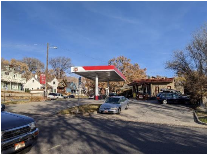
Figure 9 – West view of 860 E 3 rd Avenue.
