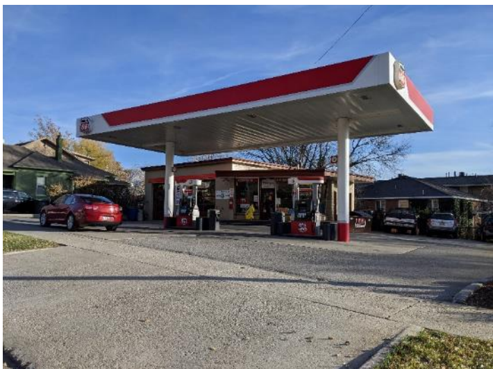
Figure 11 – Gas station and auto repair at 860 E 3 rd Avenue.
