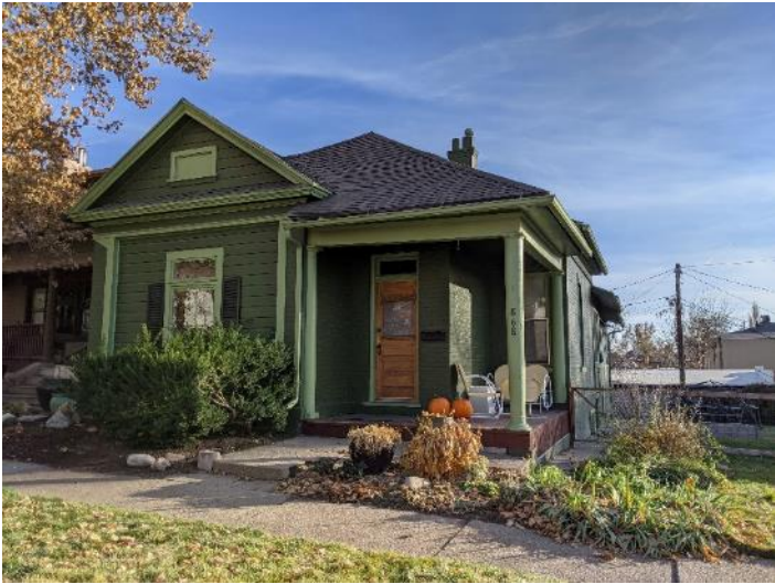
Figure 13 – House on 868 E 3 rd Avenue.
