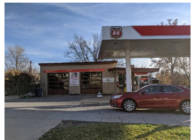
Figure 12 - Gas station and auto repair at 860 E 3 rd Avenue.
